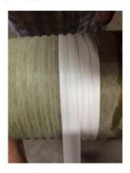
Apply two wraps (2 passes) of 1" wide Teflon tape with ½ overlap from back to front of pin. @ 450 linier inches per joint.
